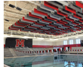
Left: Reedville Elementary School: WHISPERWAVE™ Baffles
